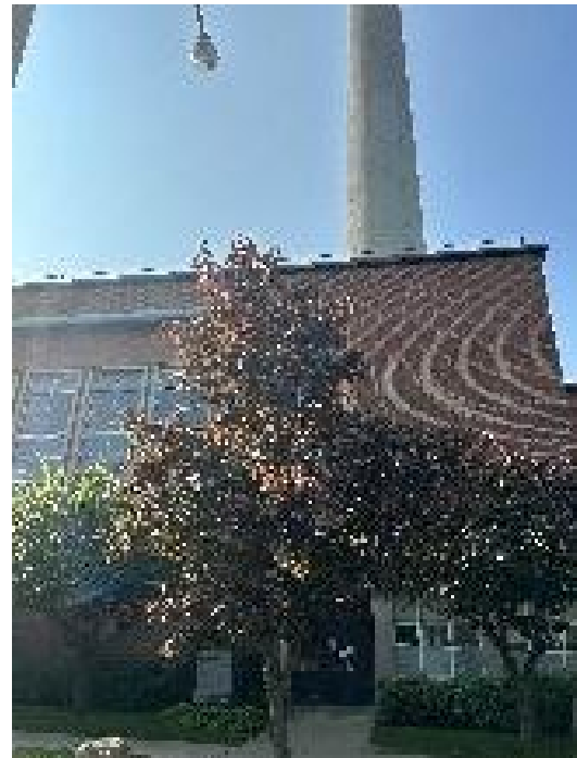
The Central Steam Plant across the street from the Burton Tower
